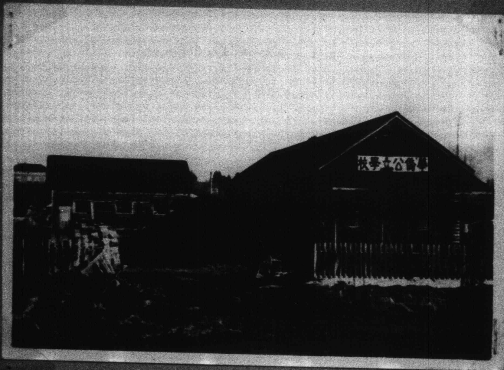
Lot 570 (School House - hall - Gym at rear)
